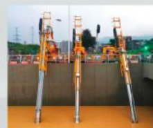
Underpass Tunnels and Culverts
