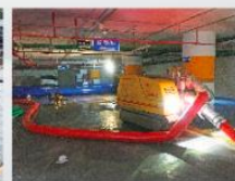
Underground Car Parks
