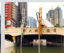
Underpass Tunnels and Culverts
